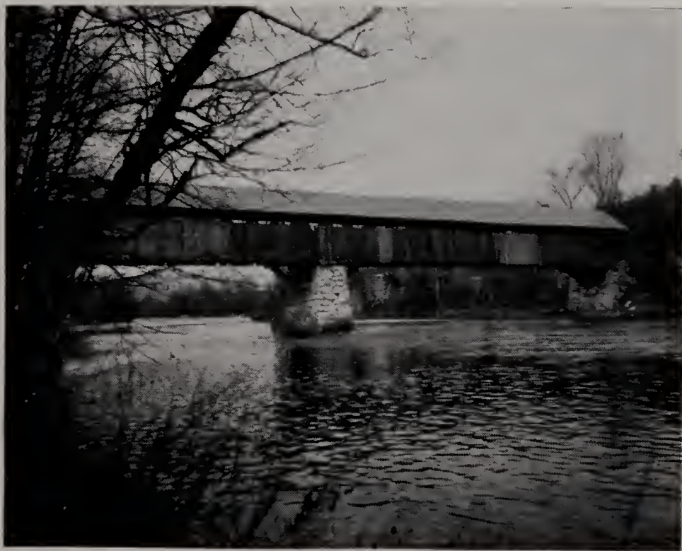
Pont Fayette, 1844–1934, over the Pemigewasset River between Plymouth and Holderness.
